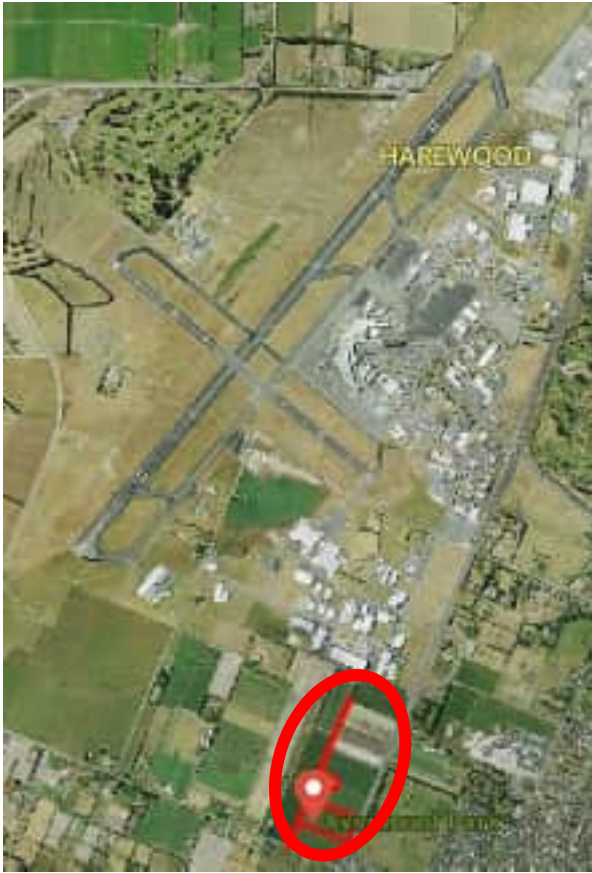
Figure 4 – proximity of the block (as indicated by the red circle) to the CIAI
